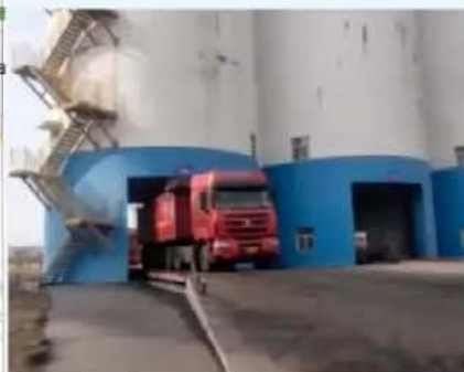
Coal mine loading silo
